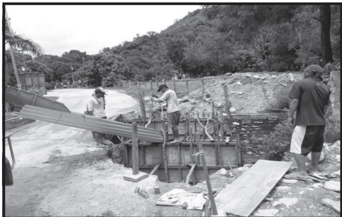
Working on the new bridge at Talipanan, Puerto Galera side
