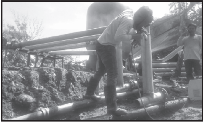
Workers installing the filtration system
